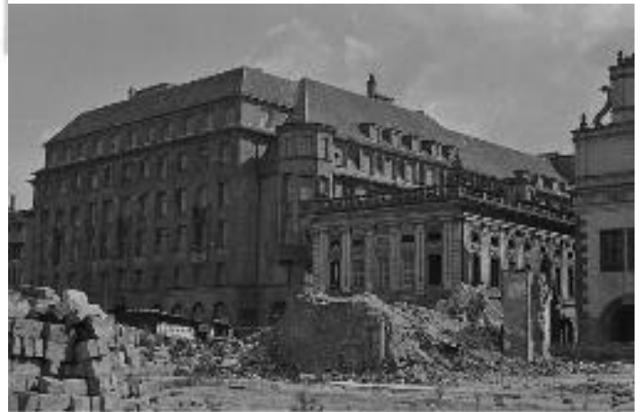
North side of the Handelshof (left), Old Trading Exchange (middle) and Old Town Hall (cut right) in 1950
