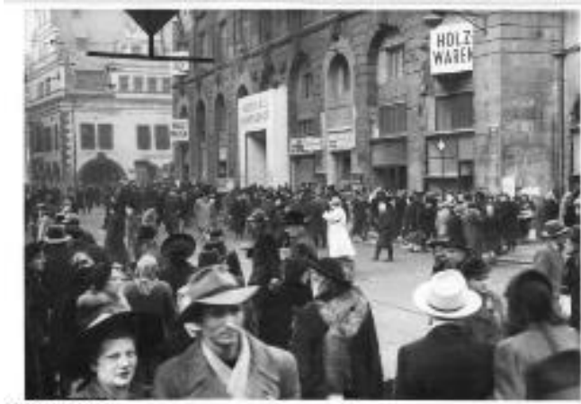
The poorly repaired facade of the Handelshof exhibition center in 1950 at the Leipzig spring fair
